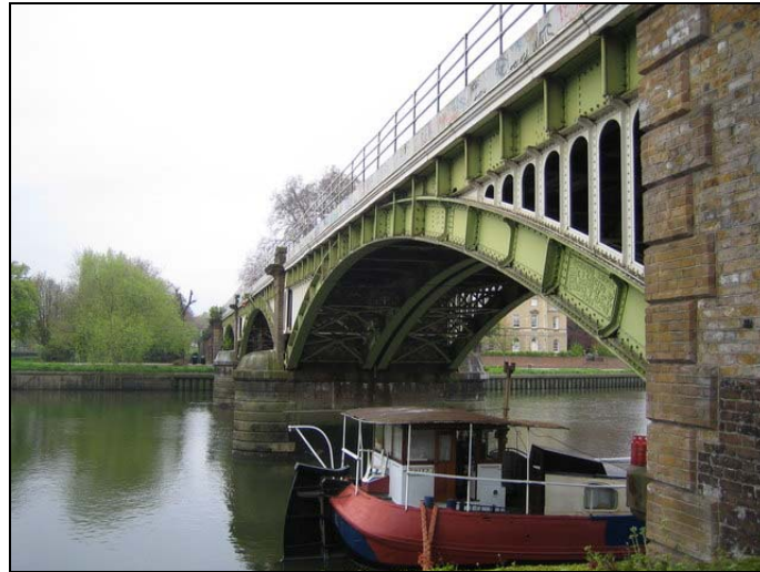
Fig 9: Richmond-upon-Thames Railway Bridge
